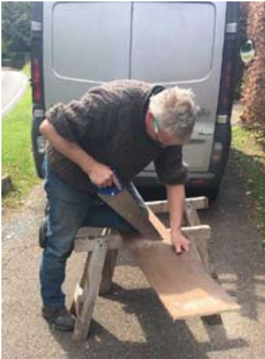
Alan Pinnock working on renovations
