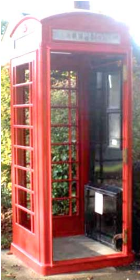
Phone Box when Renovation Started
