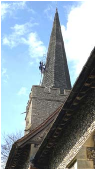
Work on the Spire (photo Gabrielle Vickery)
