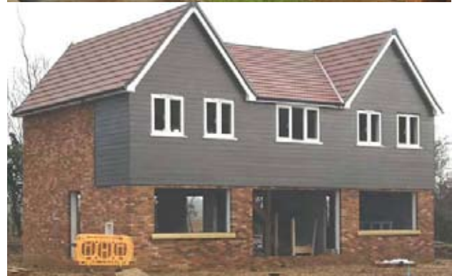
Five bedroomed house under construction
